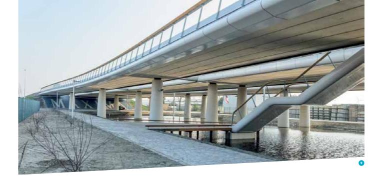
port without restrictions, beams with a length of about 100 m. The impact of this additional requirement on the structural design was minimal.
