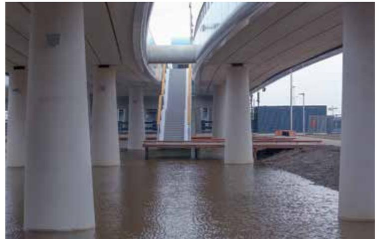
The five columns for each intermediate pier and the columns for the river piers are placed on a continuous foundation beam. At the intermediate supports, the foundation beams are supported by prefab concrete piles 450 mm square. At the river piers, steel tubes with a diameter of 610 mm are used for the foundation, in order to have enough strength to withstand a ship collision. Both prefab and steel piles are raking at 1:10. The abutments are grounded on reinforced soil constructions.
