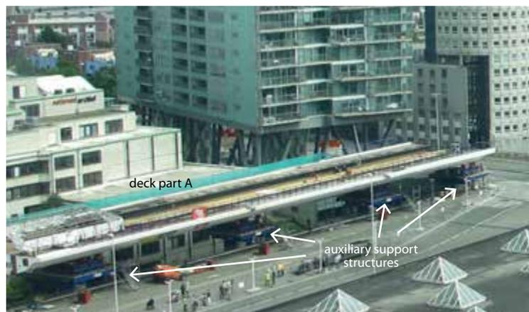
with small foundations were not capable of absorbing the summed forces from the friction and breaking forces of the metro. Also the Client did not wish an expansion joint in the railway track. Therefore the fixed point was chosen at the abutment. This choice resulted in ULS-movements of the bridge of approximately 350 mm on the other end where the platforms are located.
