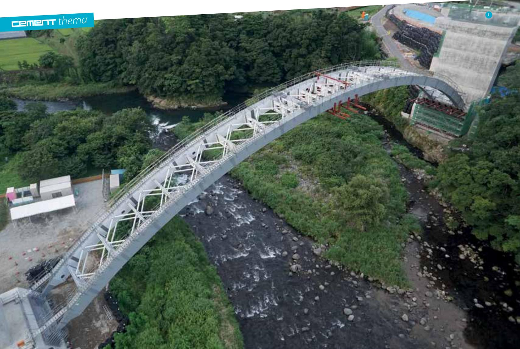
Construction of an Arch Bridge by Lowering Method
