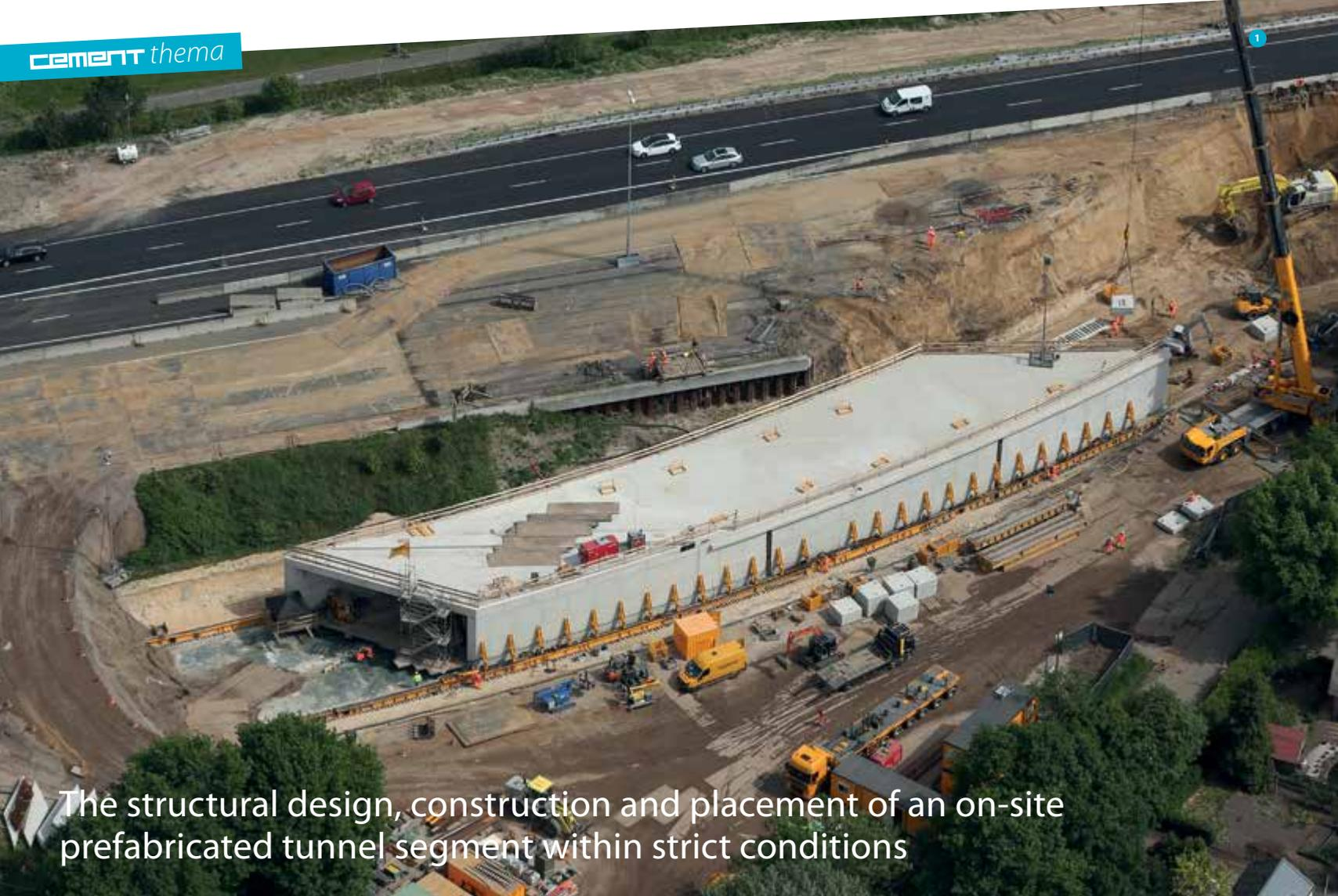
The structural design, construction and placement of an on-site prefabricated tunnel segment within strict conditions
