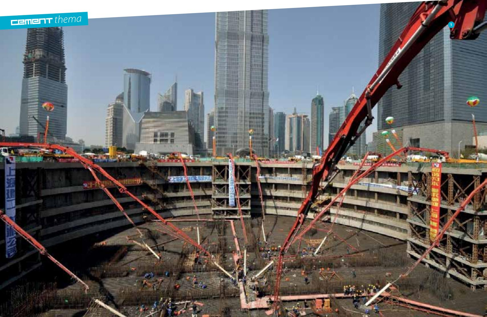
Monolithic pouring of the foundation slab of the 632 m high tower
