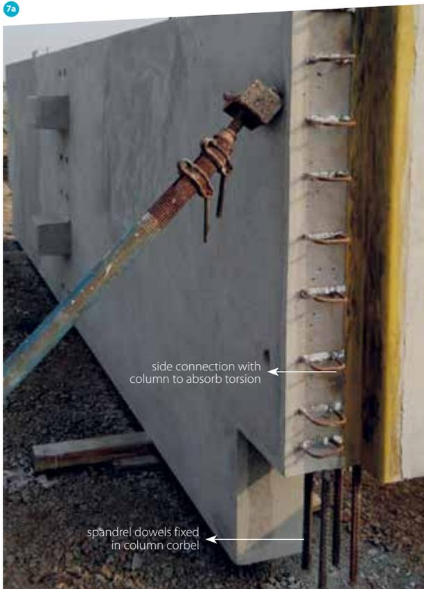
side connection with column to absorb torsion
