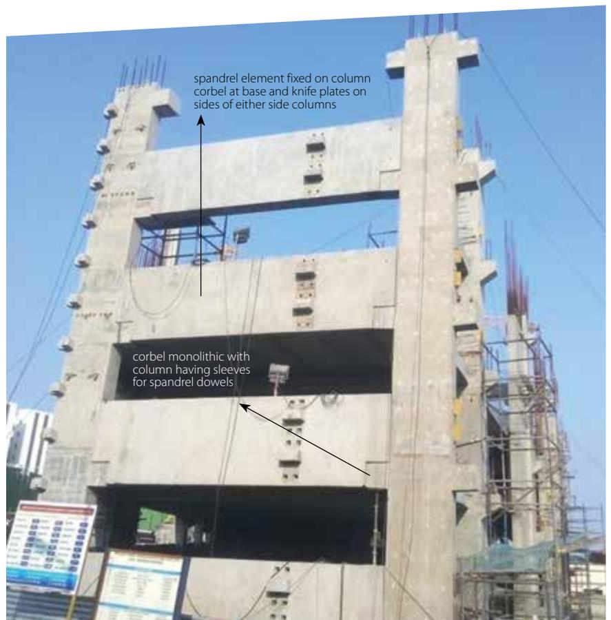
spandrel element fixed on column corbel at base and knife plates on sides of either side columns
